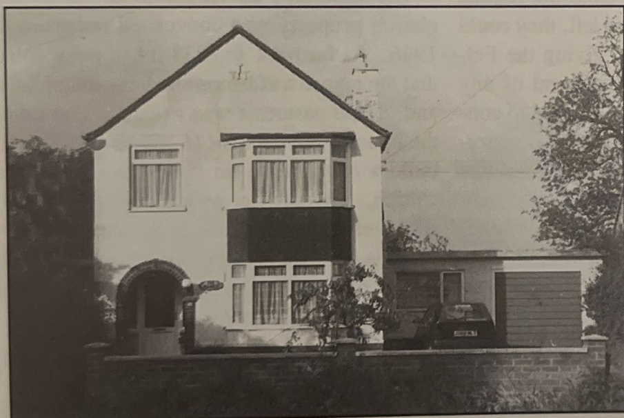
7. ...and with its newly-fitted double glazed windows and door.
