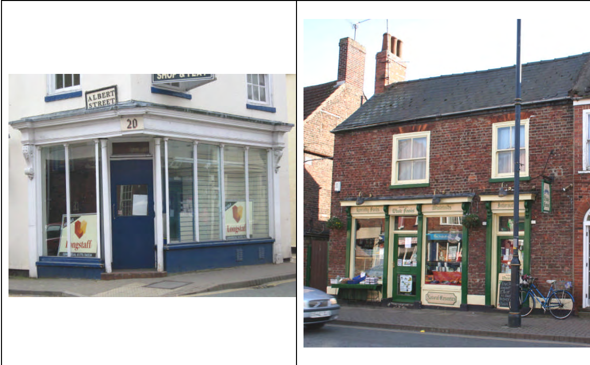
Plate 45: A pair of good historic shopfronts on High Street
