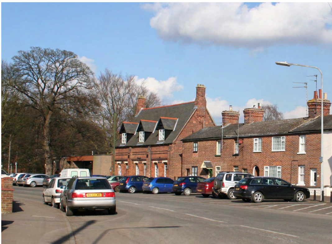
Views 7 & 8: Church Street Terrace now altered with window enlargements.
