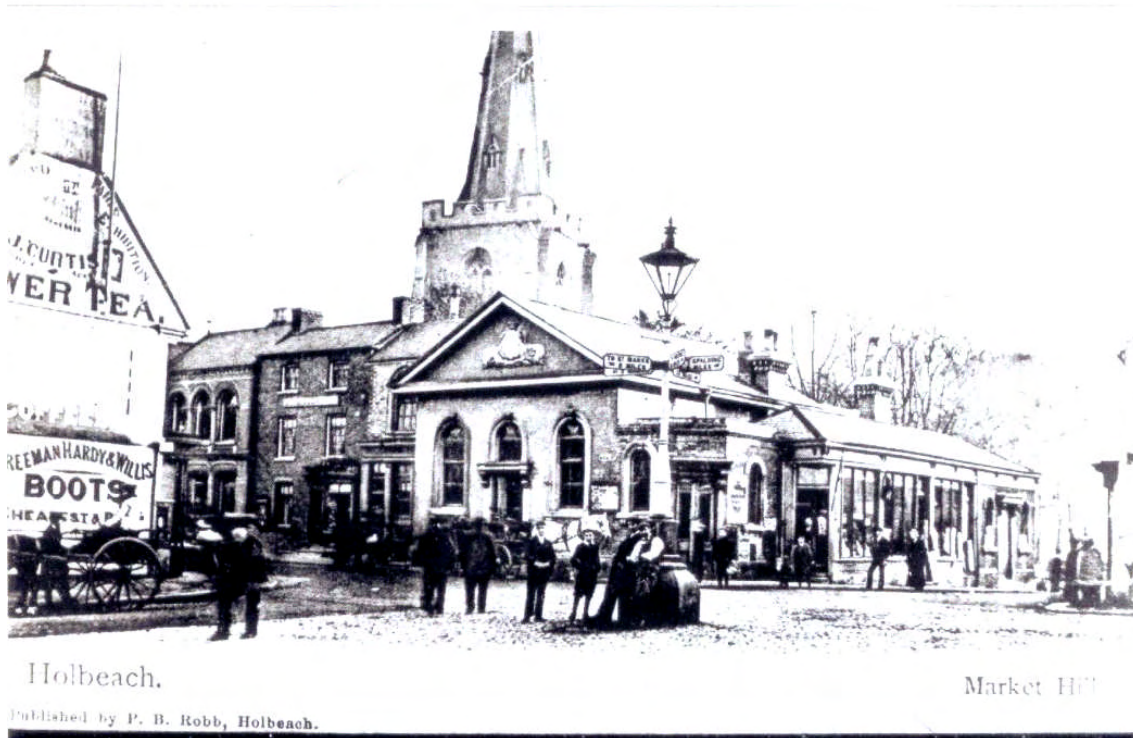
Plate 13: Market Hill showing the central feature signpost and lamp
