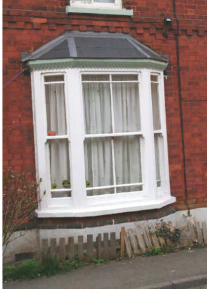
Plate 42: Attractive bay windows of Victorian properties
