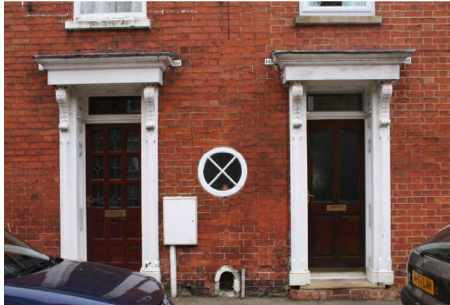
Plate 44: A pair of doorcases with hoods and central lunette and bootscraper all add interest to the facades.
