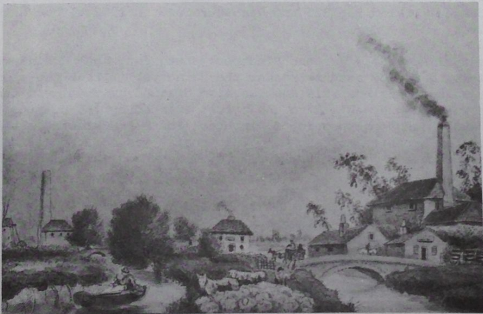
Fig.8b Pode Hole, c.1830. This shows, left to right: Wind engine and steam engine to drain Pinchbeck South Fen; the main drain of that Fen; Counter Drain with a bridge over it; and the Pode Hole pumping engines. The South Drove Drain and North Drove Drain are off the picture to the right of the engine house. See Fig. 6 and the account headed 'Pode Hole'. Hilkiah Burgess
