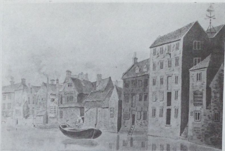
Fig.4a Warehouses at the southern end of Double Street, 1827. Hilkihah Burgess.
