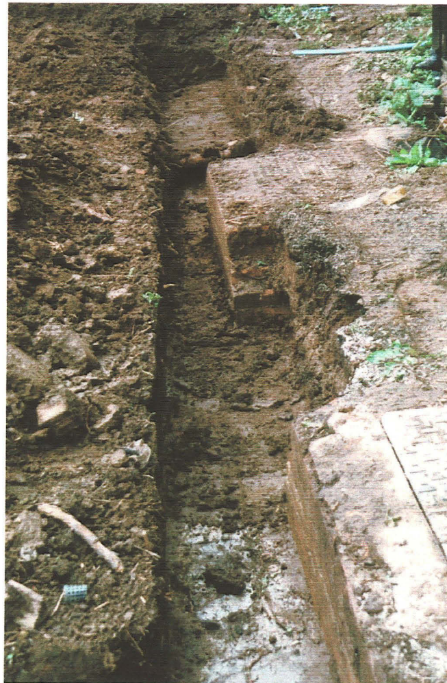
Plate 2 Western trench of development showing manholes, looking south
