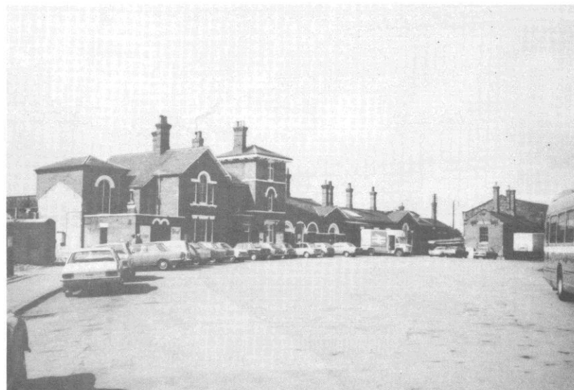
Spalding railway station 1848
