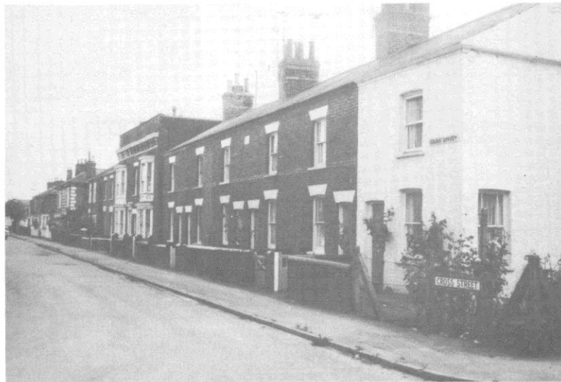
Cross Street. Post railway building. Cottages dated 1879
