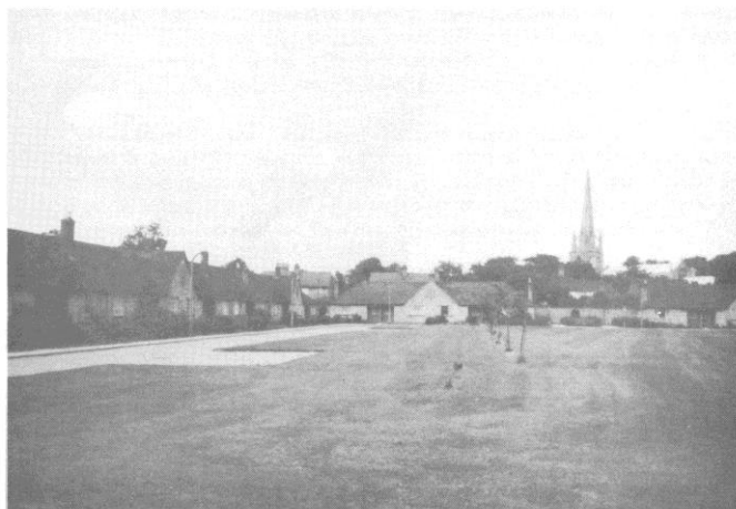
Old people's houses, Lime Court off Alexandra Road
