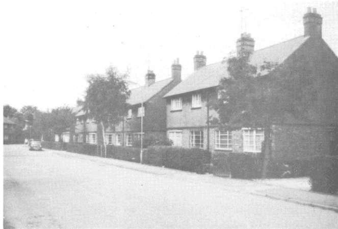
Inter-war local authority housing, Alexandra Road
