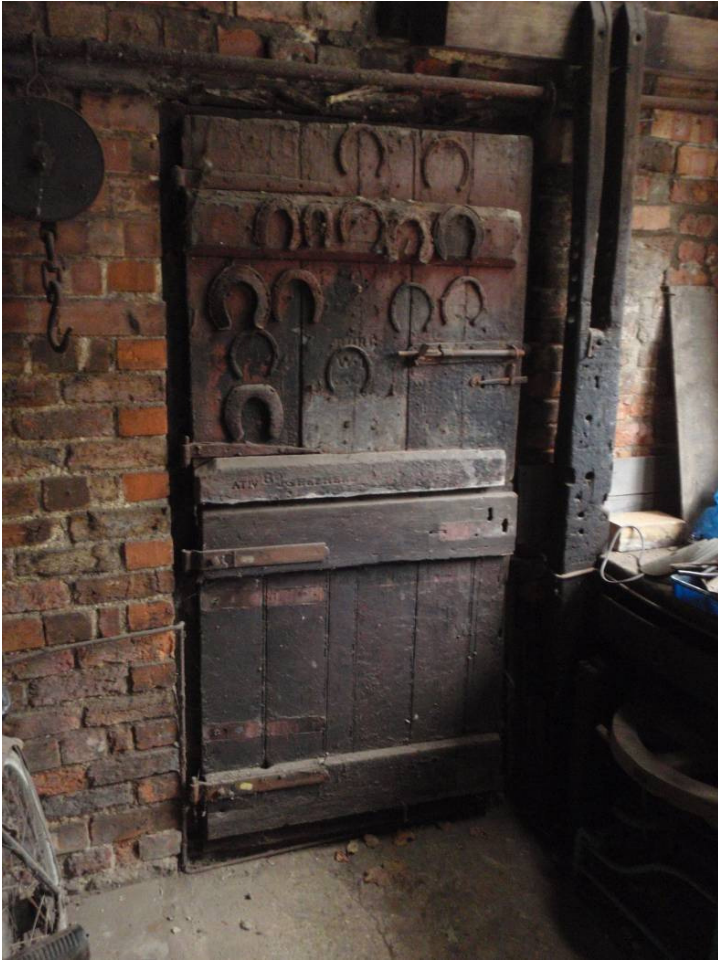
Plate 17 Door to northern room, looking northeast
