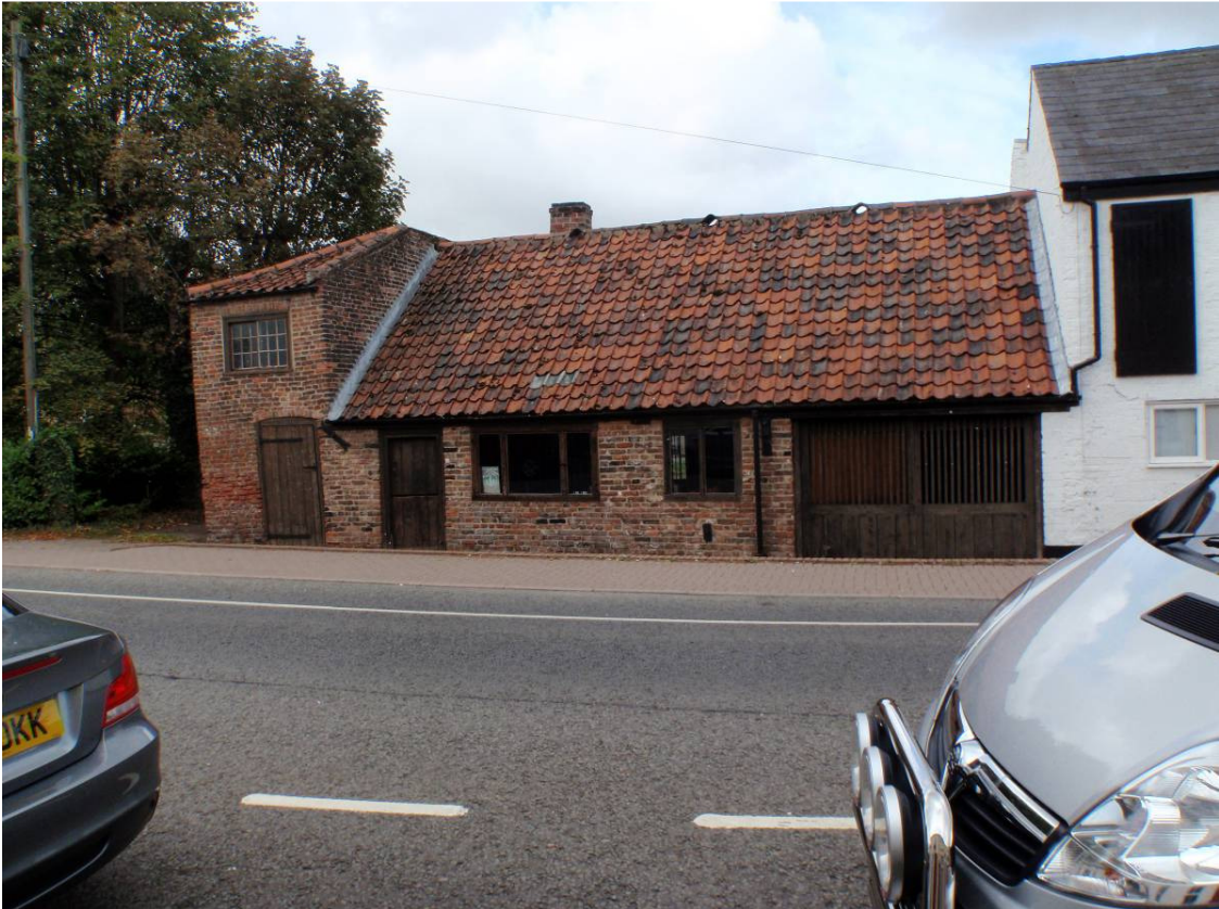
Plate 2 Eastern elevation, looking west
