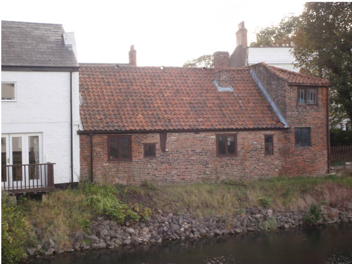
Plate 4 Western elevation, looking southeast
