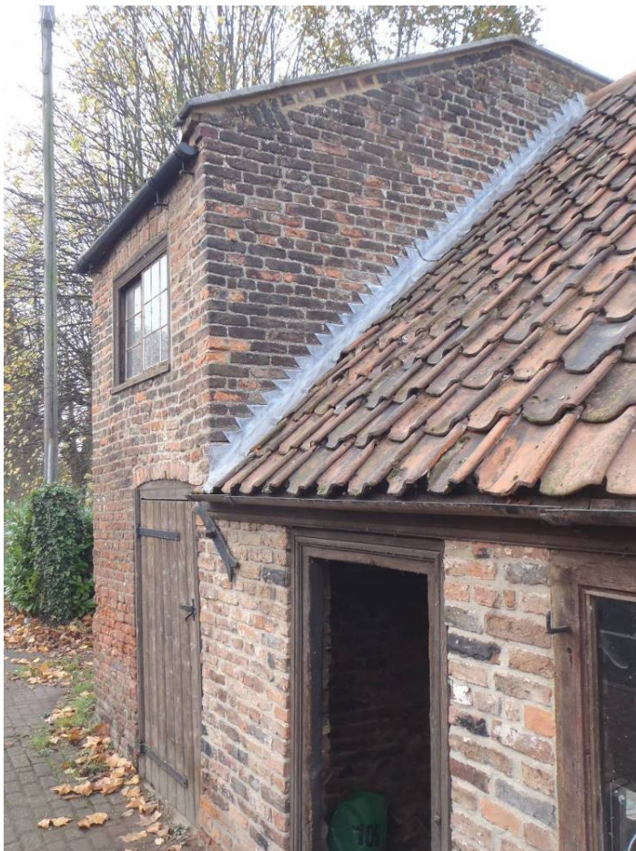
Plate 6 Detailed view, northern elevation of 2-storey block, looking southwest
