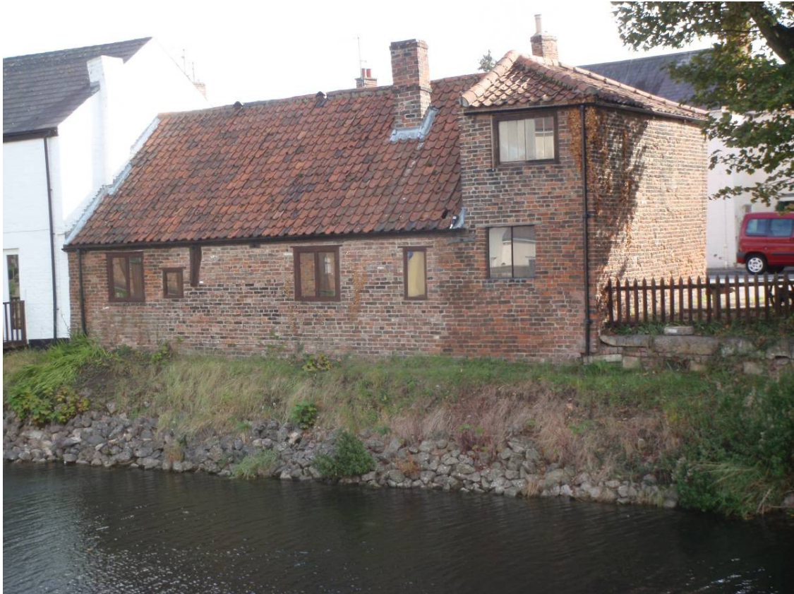
Plate 3 General view showing west and south elevations, looking east
