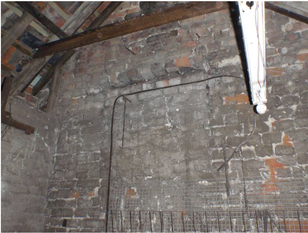
Plate 19 North wall of northern room, showing blocked window, looking north
