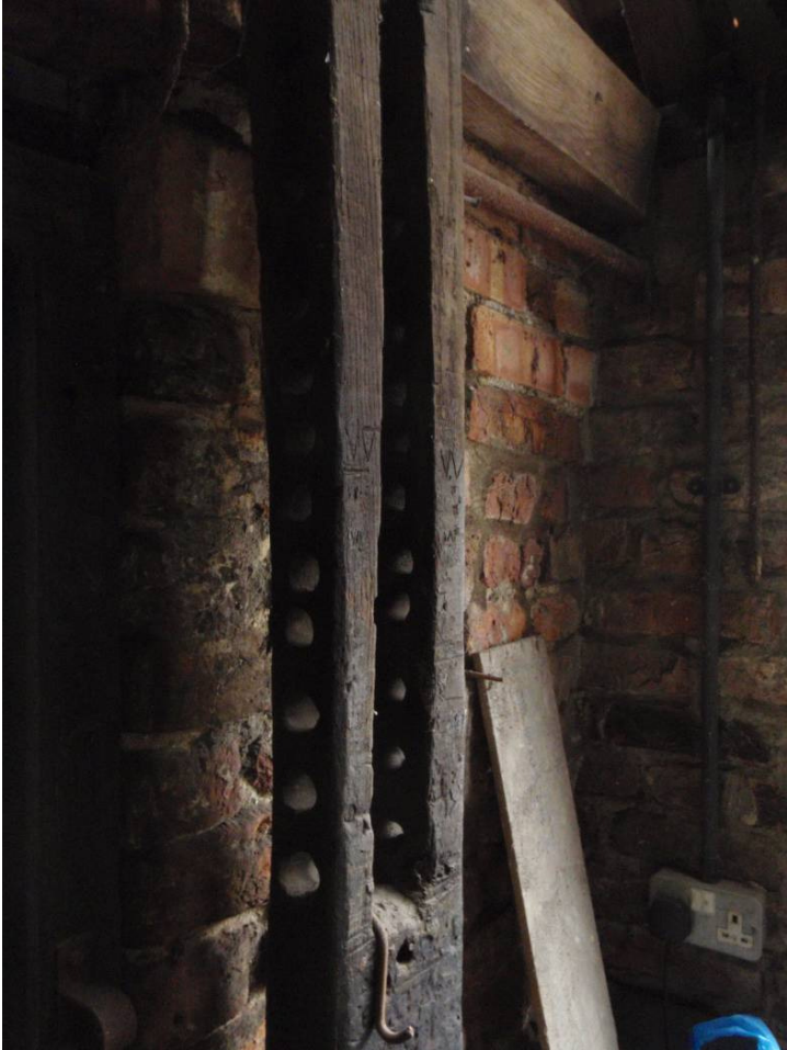
Plate 18 Detail, upright beam, showing paired drilled holes and incised 'W', looking east
