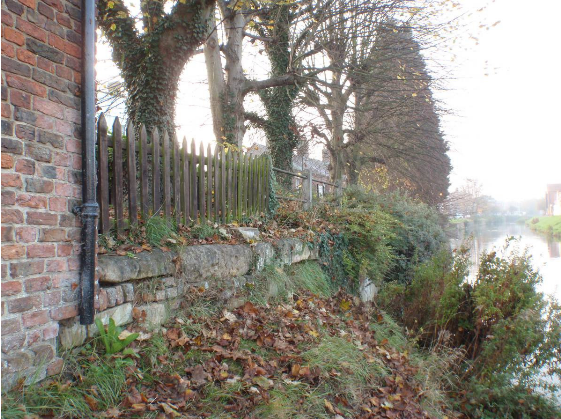
Plate 22 Section of wall adjacent to smithy building, looking south
