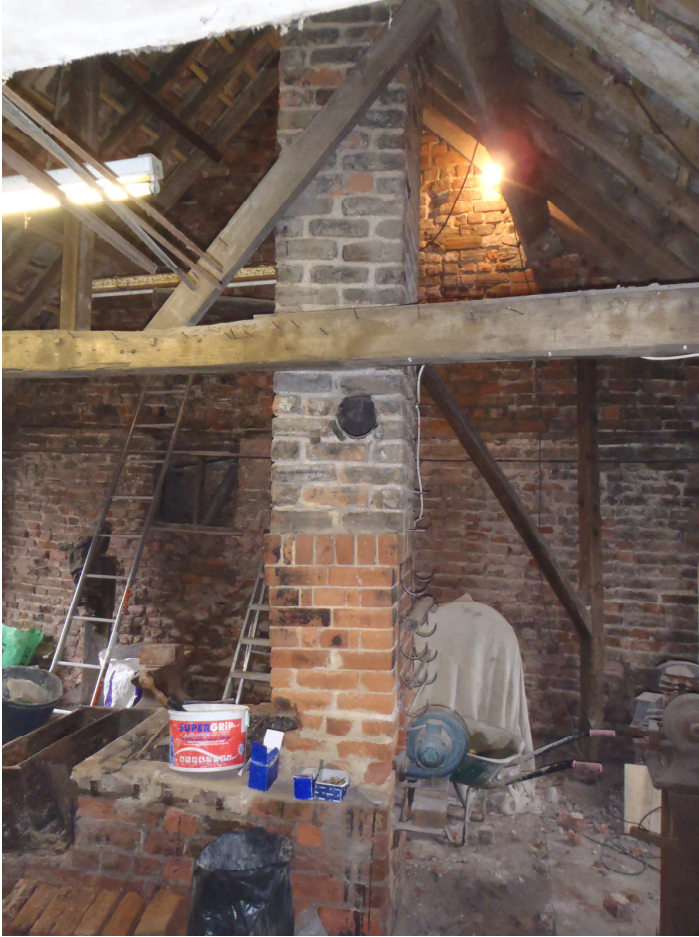
Plate 13 Forge chimney. Note rotating jib, to right of chimney, looking south
