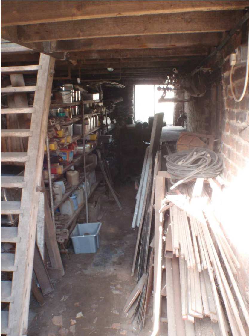
Plate 7 Two-storey southern block, ground floor, looking northwest
