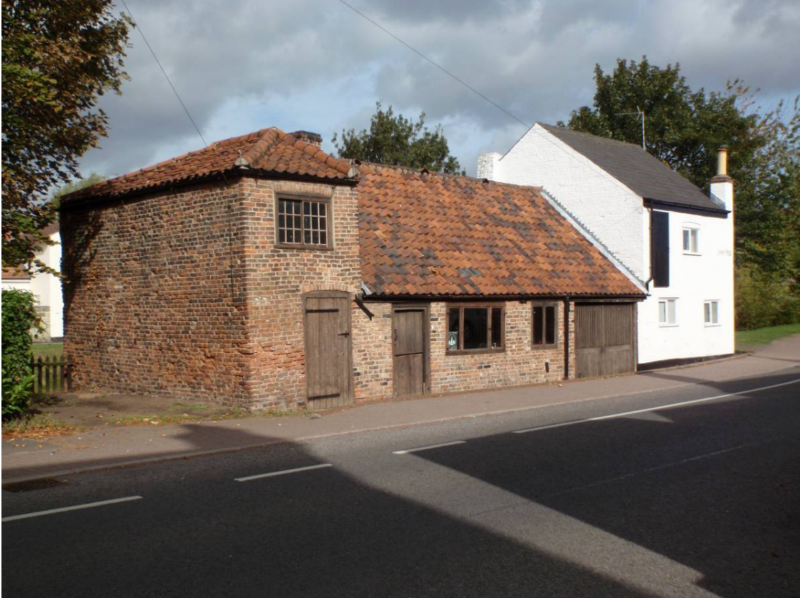
Plate 1 General view showing east and south sides, looking north
