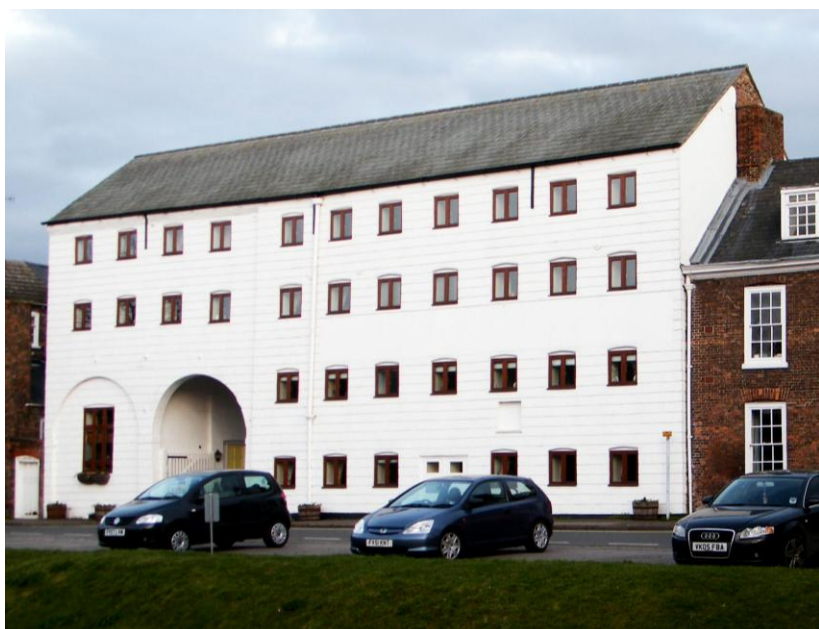
Plate 10 Converted warehouse with the bank of the River Welland in the foreground
